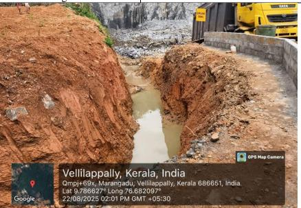
1.7 Overflow water from the siltation pond should be discharged to the nearby natural drain after adequate filtration.
